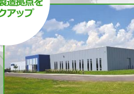
Moriroku Technology North America Head Office & R&D
